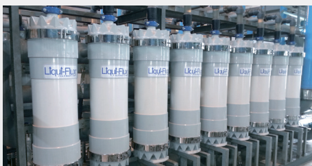
Process Water Power Plant | 240m 3 /h
