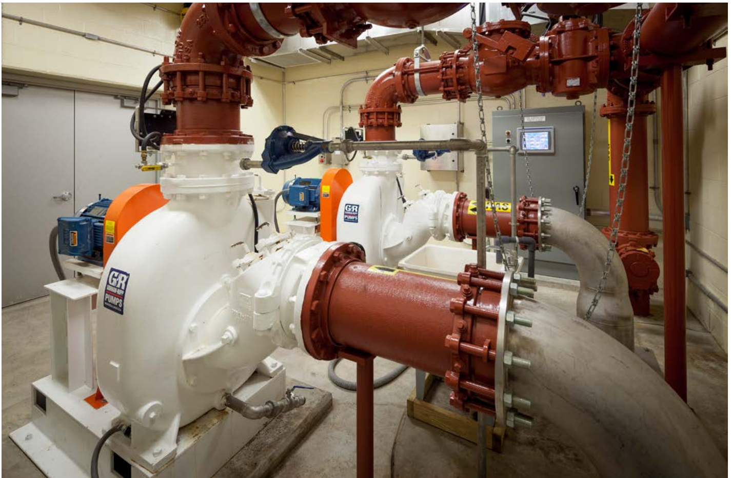
10" Super T Series® return activated sludge (RAS) pumps
