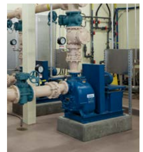
Super T Series® dewatering feed pumps
