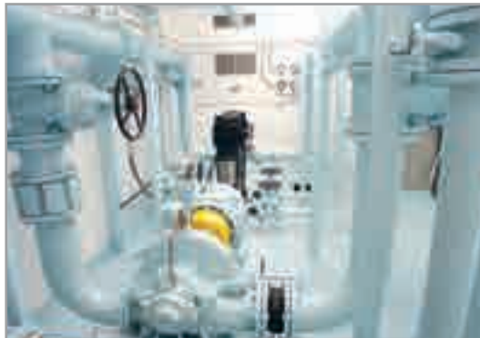
Above Ground Installation.
