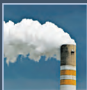
AIR POLLUTION CONTROL
