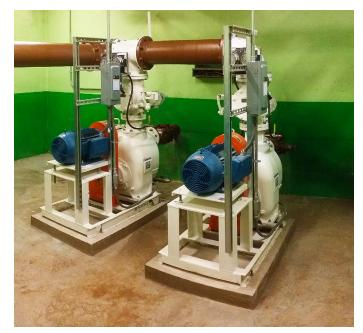
Gorman-Rupp Super T Series® pumps can be mounted above the liquid being pumped. Should service or maintenance be required, it can be easily performed using common hand tools and without disconnecting piping.
